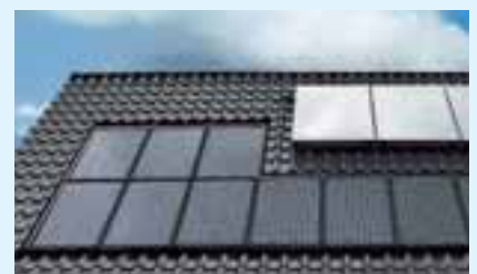
New photovoltaic modules give the appearance of a continuous surface (top right), unlike conventional systems (bottom).
