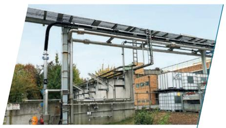
sure." It's also been reinforced with special arches that act like a spring. If the black wastewater pipe expands in the sunlight, it can therefore yield without the risk of distortion, which would cause undesirable inner tension. The wastewater pipeline is only routed underground for the final section, from the microbiology facility to the wastewater treatment plant. Supply Center Bergkamen uses rainwater for operational purposes
